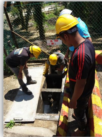
The workers are being trained how to use drip tray (left) and oil trap (right).
