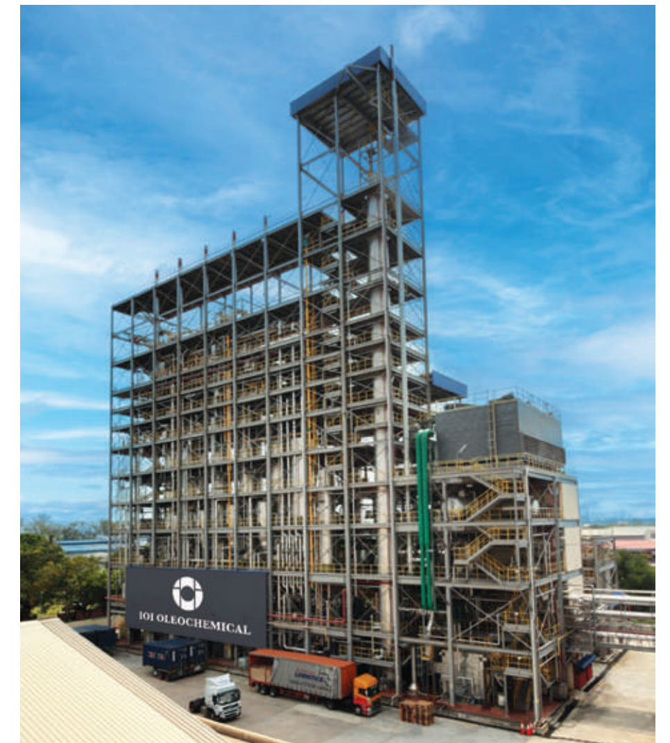
Our new oleochemical plant in Prai, Penang with a capacity of 110,000 MT per year.
