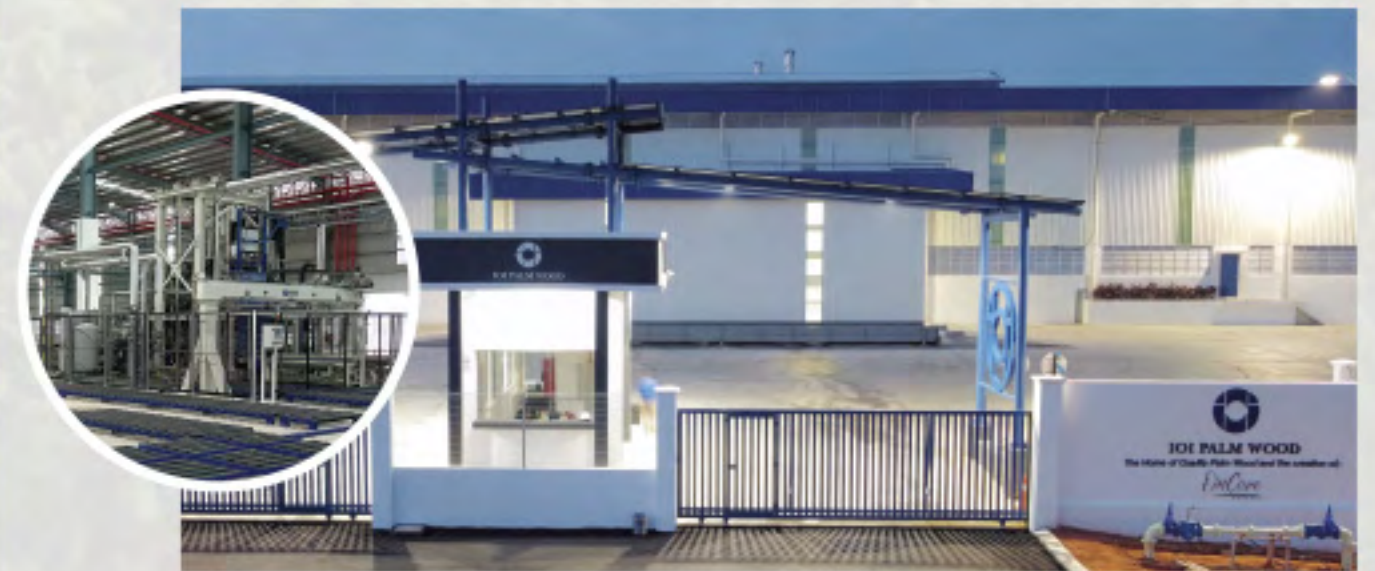
IOI's new Palm Wood Manufacturing facility in Johor
