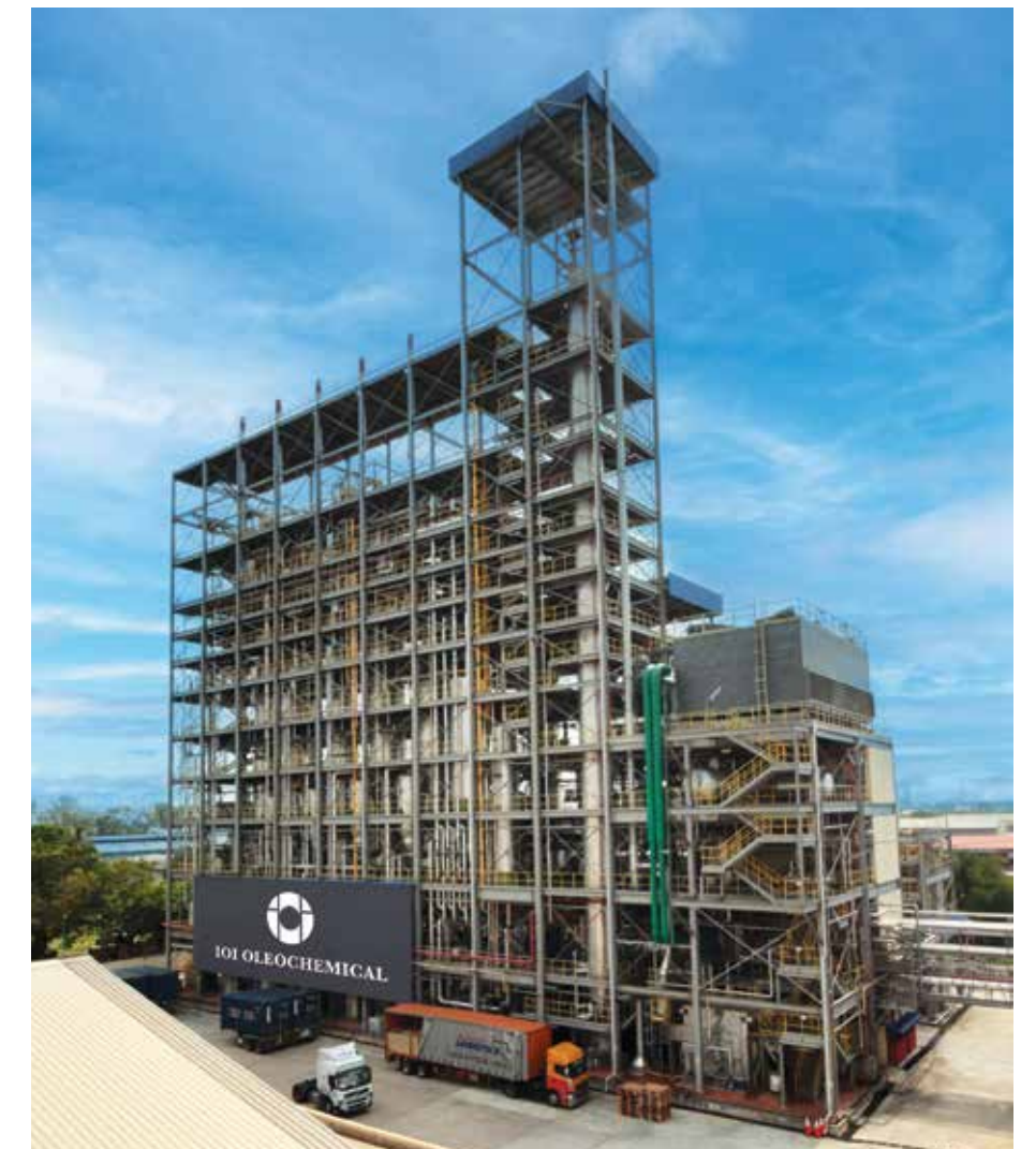
Our new oleochemical plant in Prai, Penang with a capacity of 110,000 MT per year.
