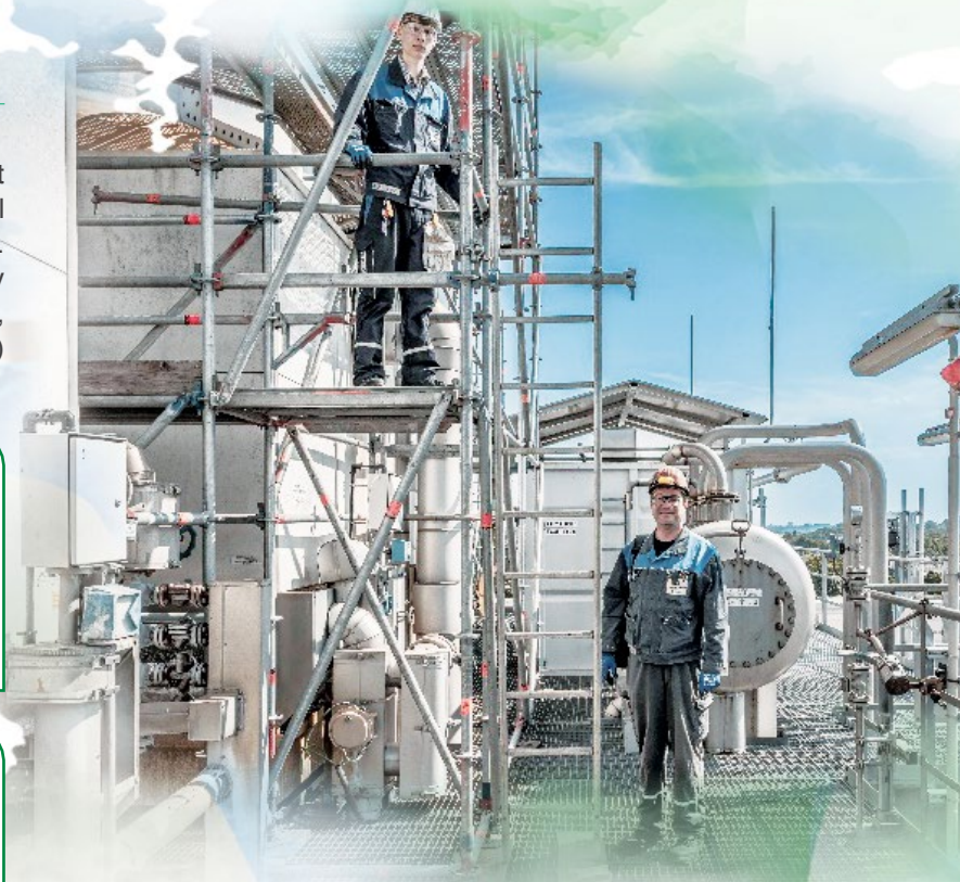
IOI employees inspecting one of our Oleochemical facilities in Germany
